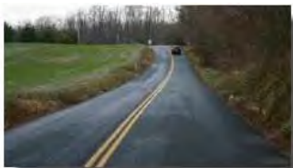
Centerline for No Passing on horizontal curve.
