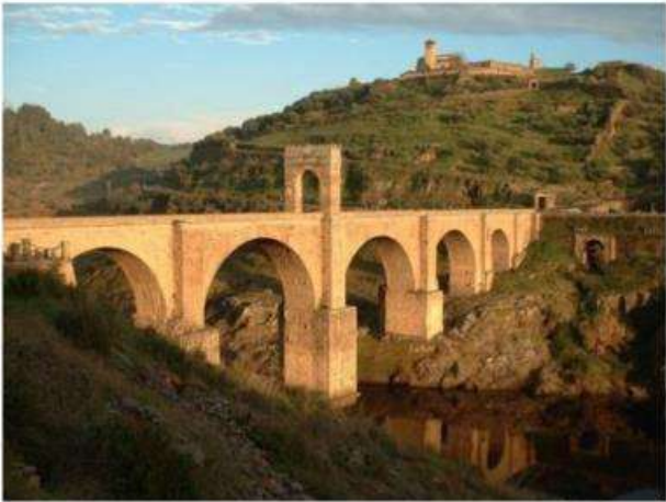
Figure 1. Roman Alcantara Arch Bridge in Spain
