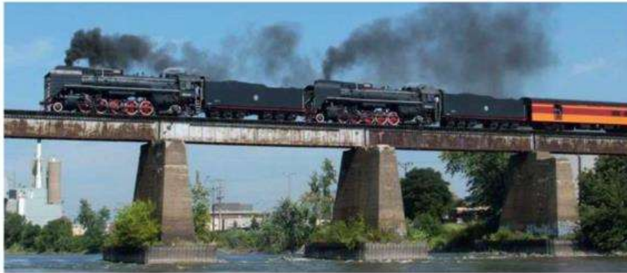
Figure 3. Example of a steel beam bridge
