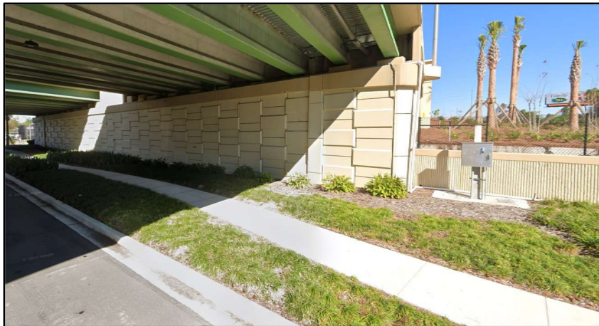
Figure 3: Finished MSE Wall After Widening (Source: Google Street View)
