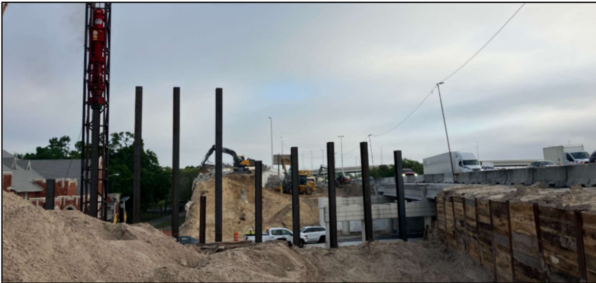
Figure 1: Widening of Existing Bridge
