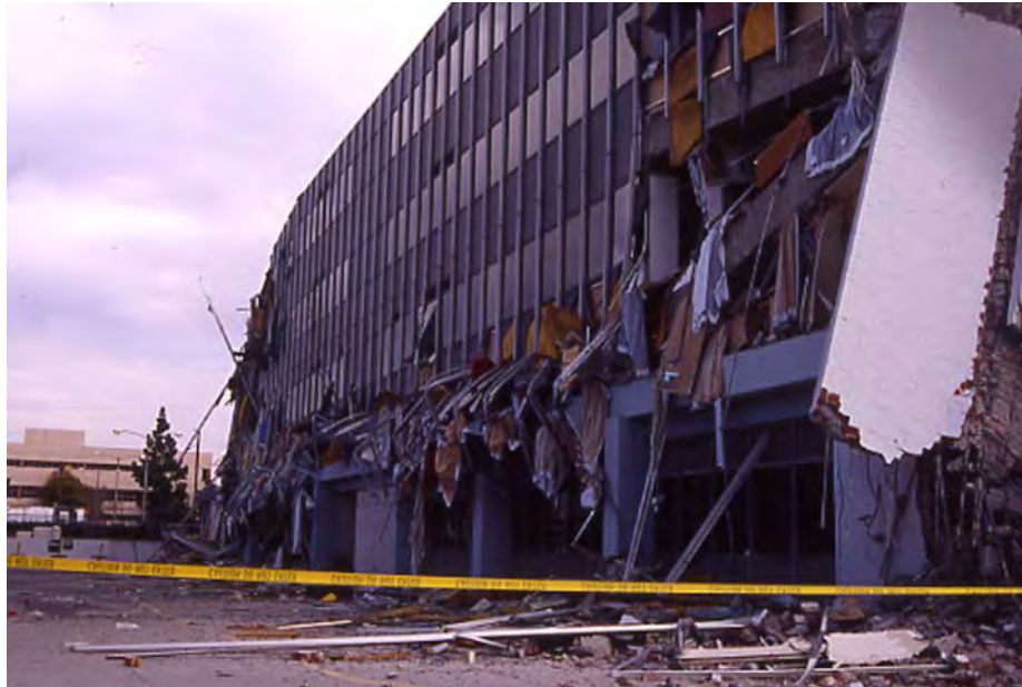
Figure 6-2 Exterior view of medical office building severely damaged by the 1994 Northridge earthquake. (C. Arnold photo)
