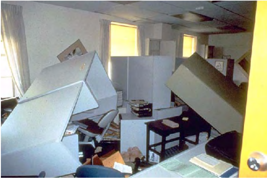
Figure 6-1 Typical earthquake damage to contents and nonstructural components in a modern office building. (photo courtesy of the Earthquake Engineering Research Institute)
