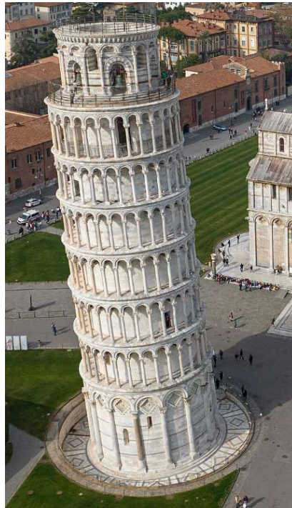
Fig. 2- The Leaning Tower of Pisa
