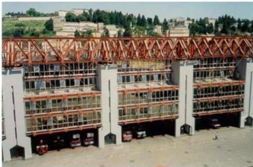
Fig. 4. The first seismically isolated fire-command building in Naples, Italy
