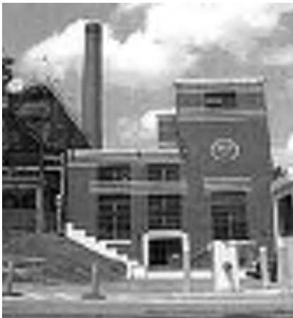
Figure 1. The NIOSH boiler plant was modified to cofire biomass with coal.
