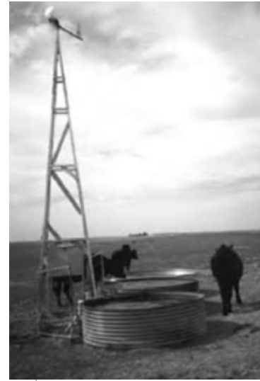
This 1-kW Whisper turbine provides direct AC power for the water pump for stock tanks on a ranch in Wheeler, Texas.
