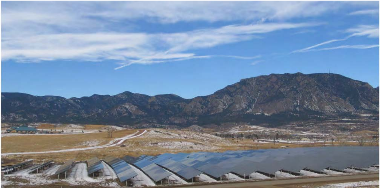
Figure 2. Fixed tilt PV solar array at Fort Carson, CO
