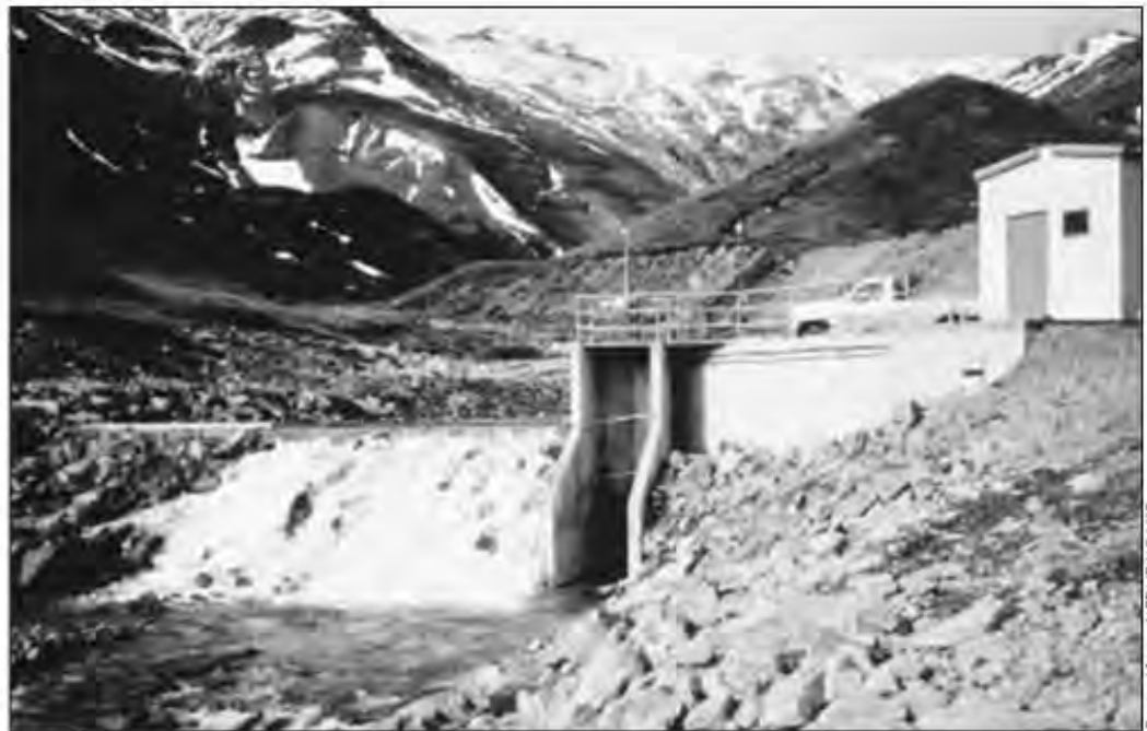
This small-scale hydropower system is helping an Alaskan community save money on their electricity.
