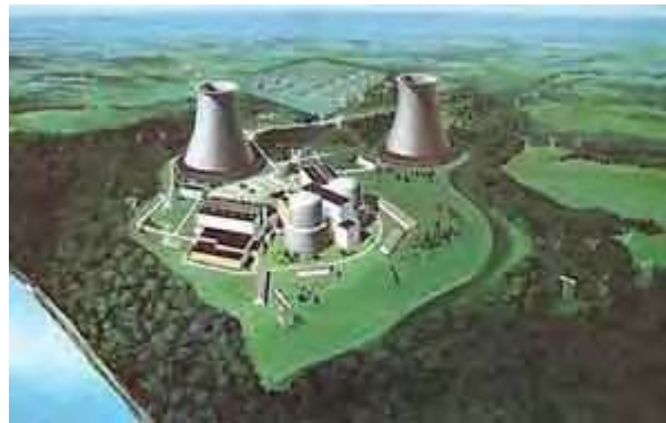
Figure 2 - A complex project such as a nuclear power plant is required by federal law to have a comprehensive QA program that addresses all 18 criteria. However, the principles of QA are applicable to and beneficial for all types and sizes of projects dealing with the design and construction of structures, the manufacturing of products and the performance of professional services.
