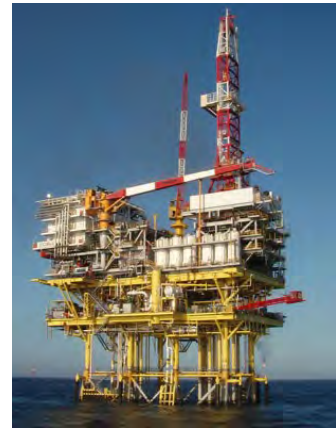
Figure 5: Fixed Drilling Platforms
