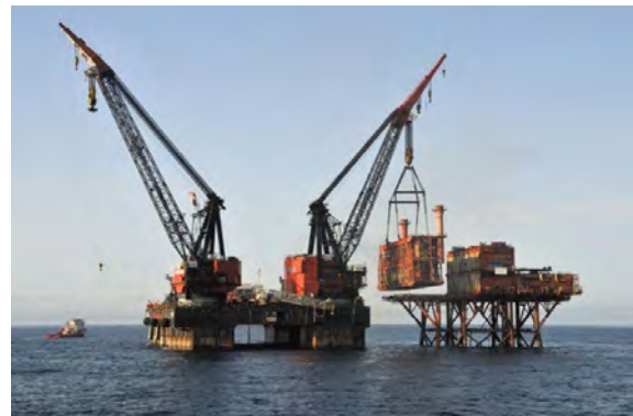
Figure 1: Decommissioning in operation
