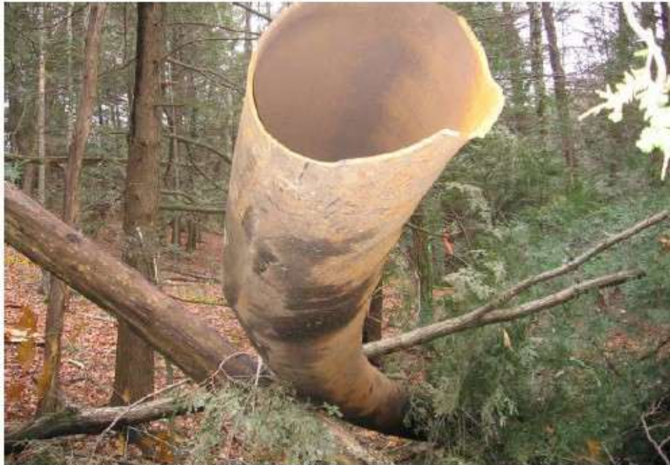
Figure 7: Bent 21.7 foot section of pipe in swamp
