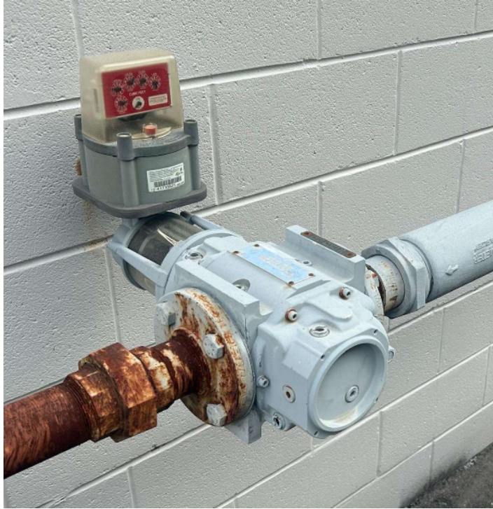
Figure 1 - A rotary meter supplying gas to my local grocery store. Source: Robert Noriega (self)
