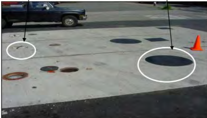
View of sump lids
