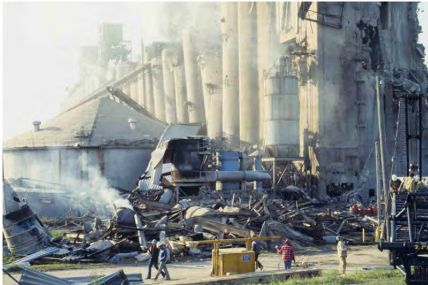
Figure 1 – Aftermath of grain elevator explosion, Westwego, LA
