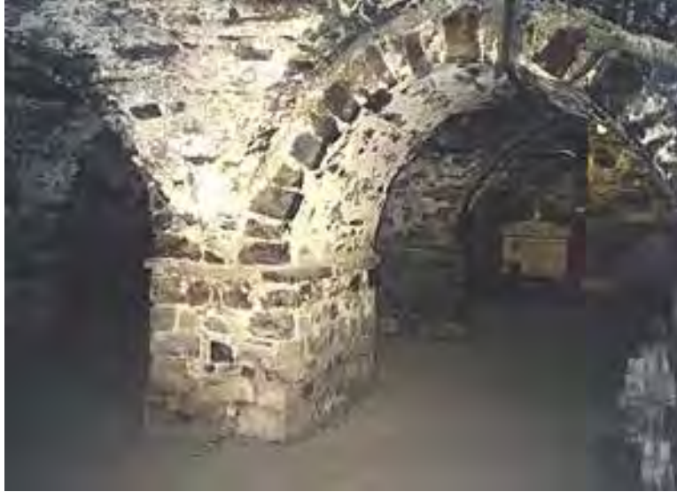
Photograph 1.1 - Foundations for a Medieval Era Cathedral
