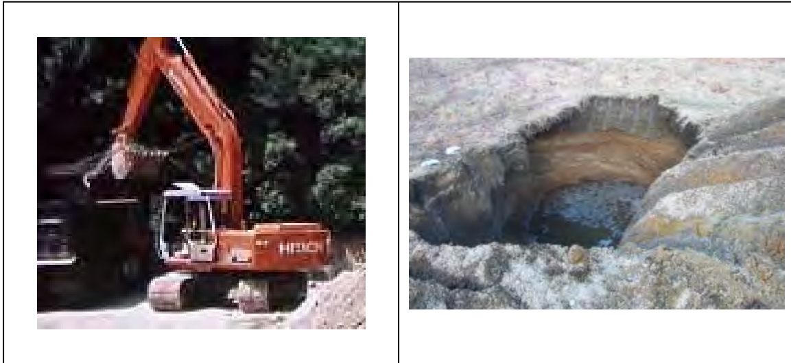
Photograph 2.1 – Test Pit Excavation
