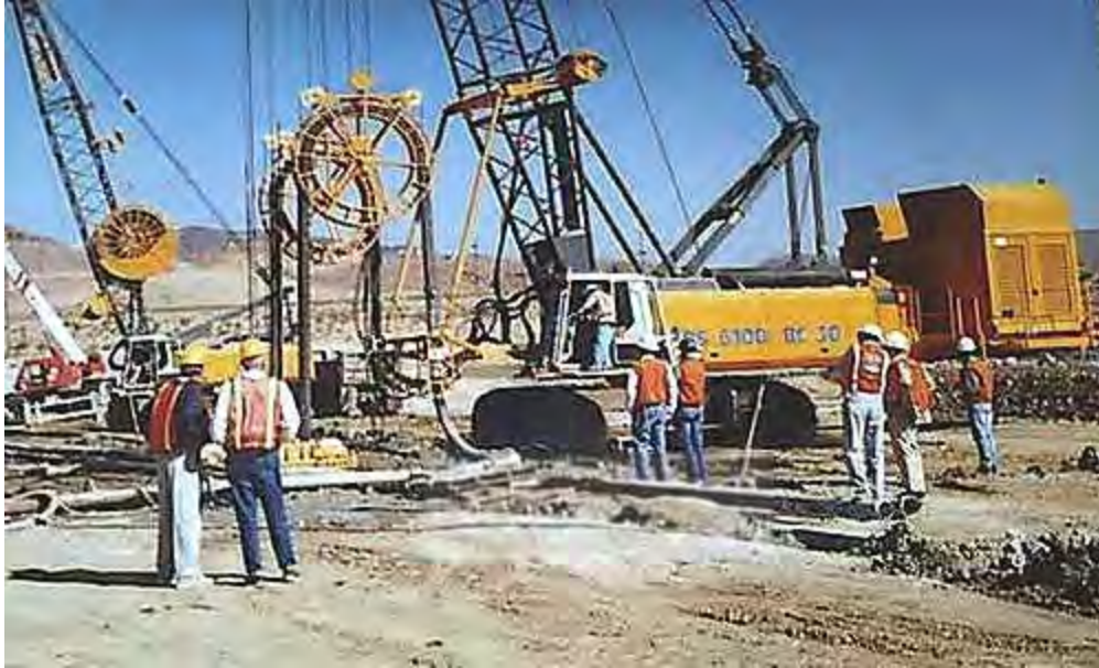
Figure 2: Example of the type of heavy track-mounted equipment that needs special handling to get on site and assemble for use. This equipment was operated to dig and install a cut-off wall in the foundation of a major dam.
