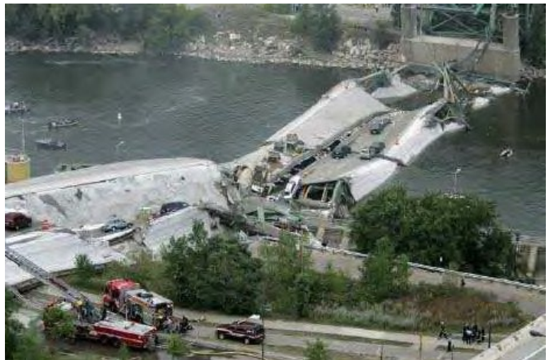
Figure 2: Collapsed north section of bridge. (Source: NTSB.)
