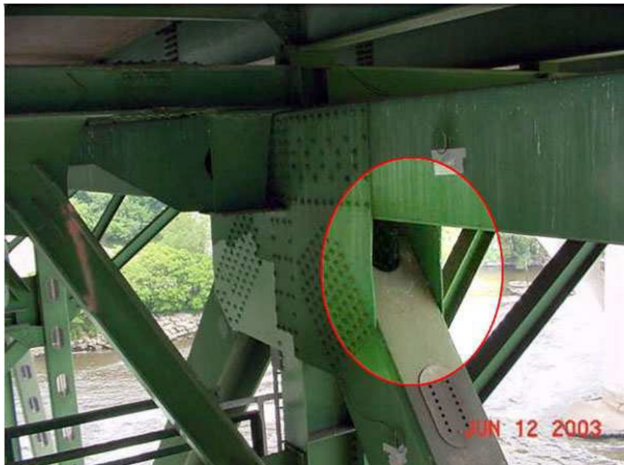
Figure 3: Bowed and significantly distorted gusset plate. (Source: NTSB.)
