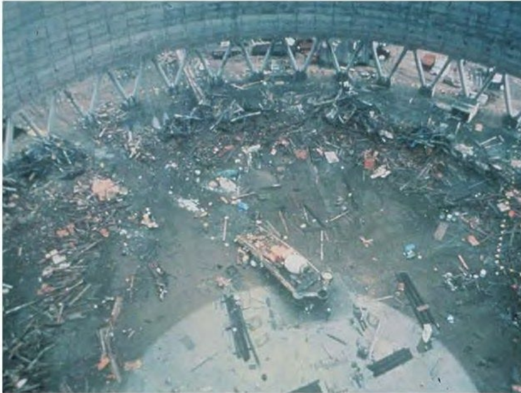
Figure 2 – Cooling Tower Collapse Aftermath
