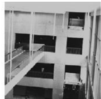
Figure 1. Third Floor Walkway (left)
