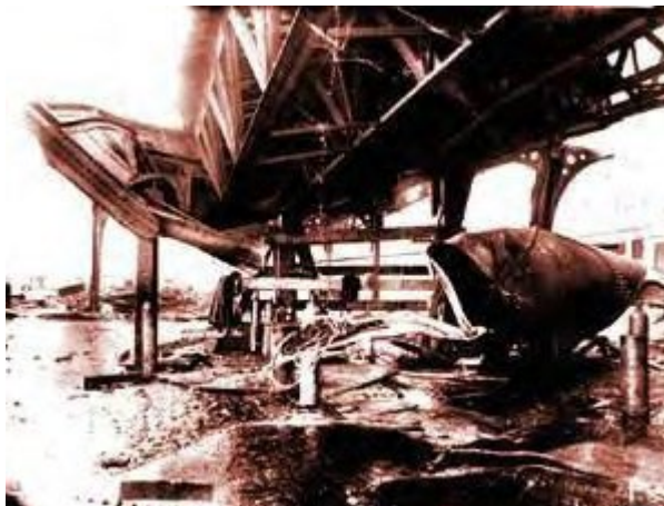
Elevated Rail after the Flood
