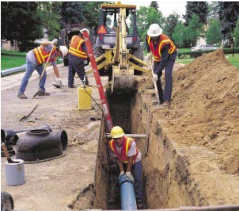
Water main maintenance. Photo by the American Water Works Association.
