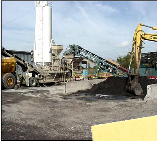
Figure 3-2. Ex-Situ Soil Remediation at Peak Oil Site
