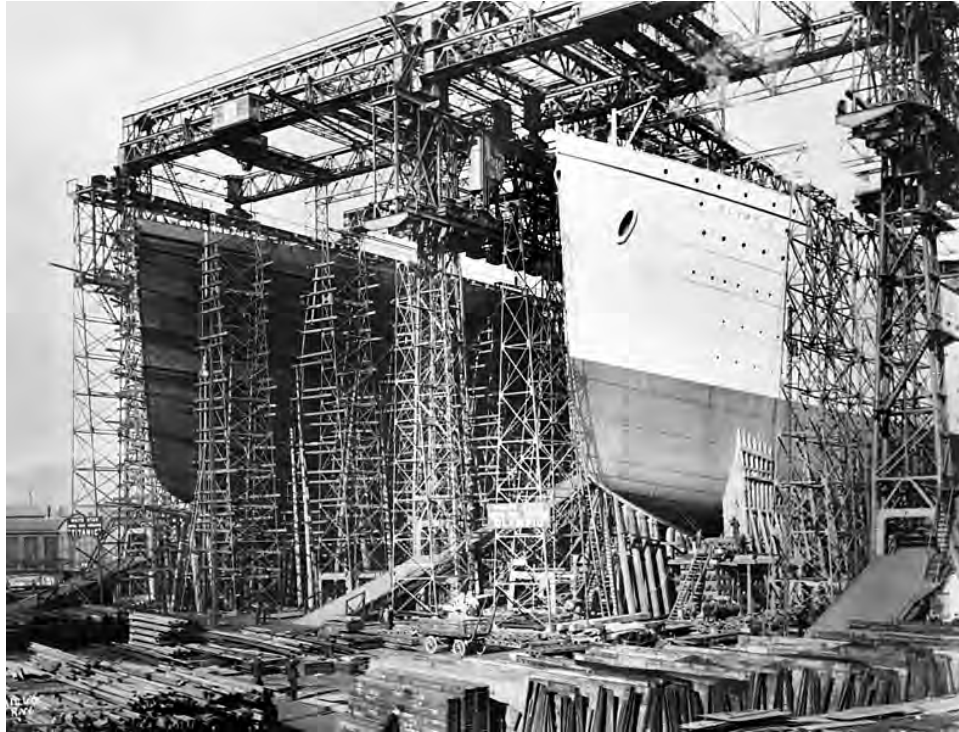
Figure 3. The Titanic (left) and the Olympic (right) were built in parallel by Harland and Wolff in their dry docks in Belfast, Ireland. A part of the large gantry system is also visible. Large steel plates used in the hull are visible in the foreground.
