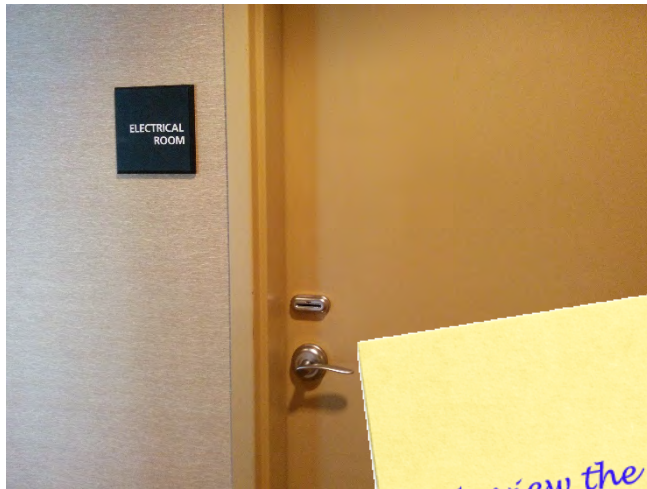
Accessible electrical equipment behind locked door
