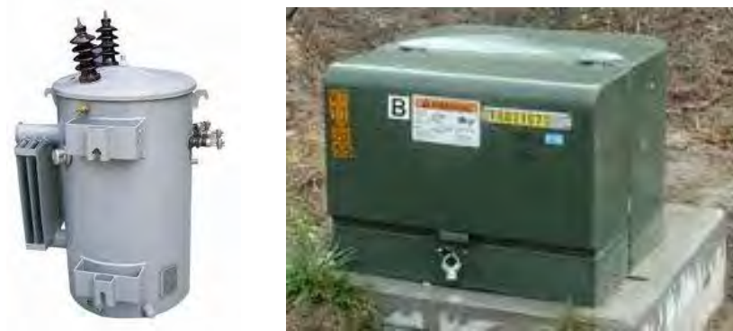
Figure 2.2 Pictures of Pole Mounted and Pad Mounted Single Phase Transformers
