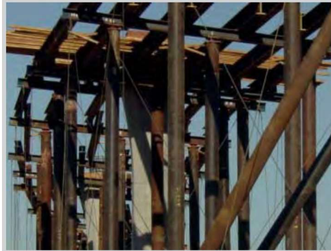
Figure 2- Typical falsework for this project
