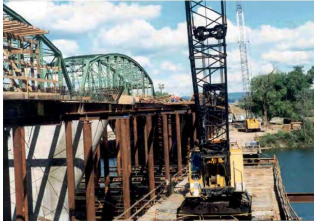
Figure 1 - Pipe Post Falsework
