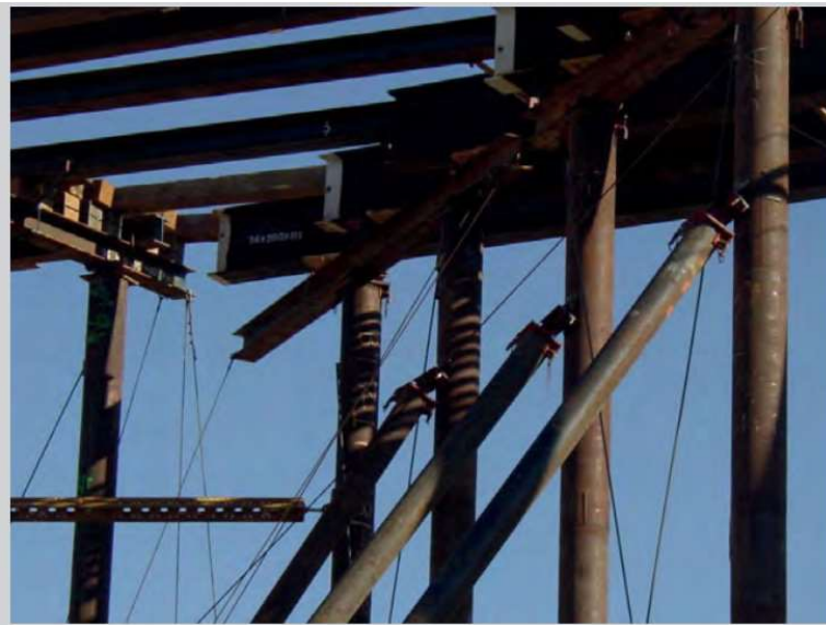
Figure 3- Push-pull braces added to falsework.
