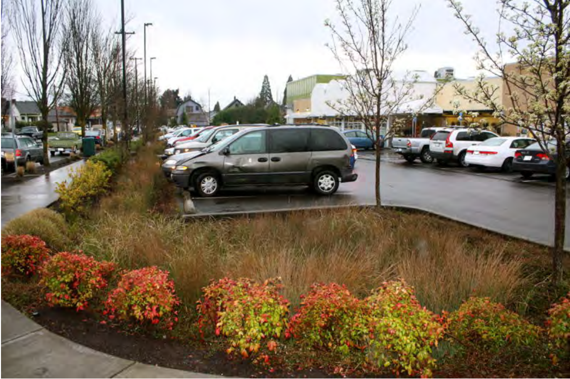
Figure 1 – Bioretention Cell adjacent to a parking lot
