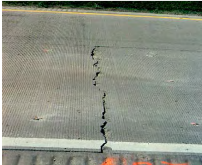
Figure 1. Transverse crack
