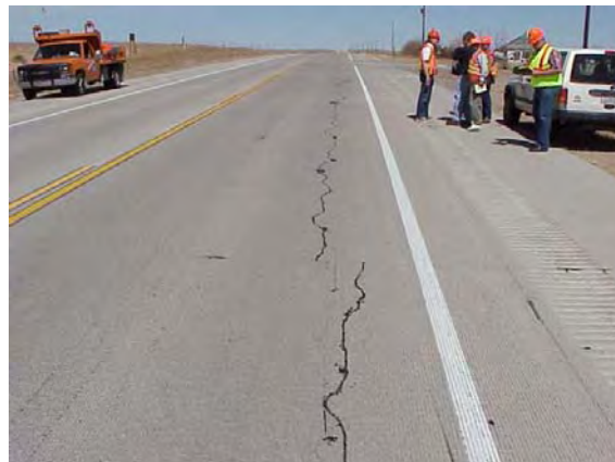
Figure 2. Longitudinal crack
