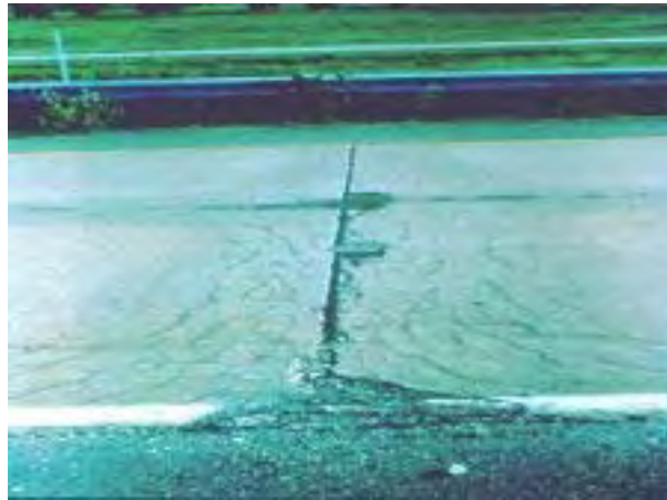
Figure 3. "D" cracking
