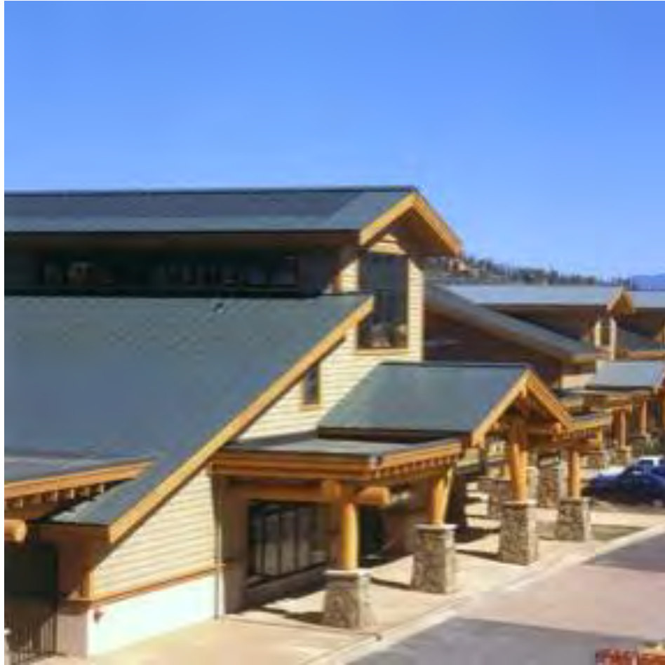
(Bighorn home improvement center in Silverthorne, Colorado and an example of daylighting. Photo Courtesy: DOE)
