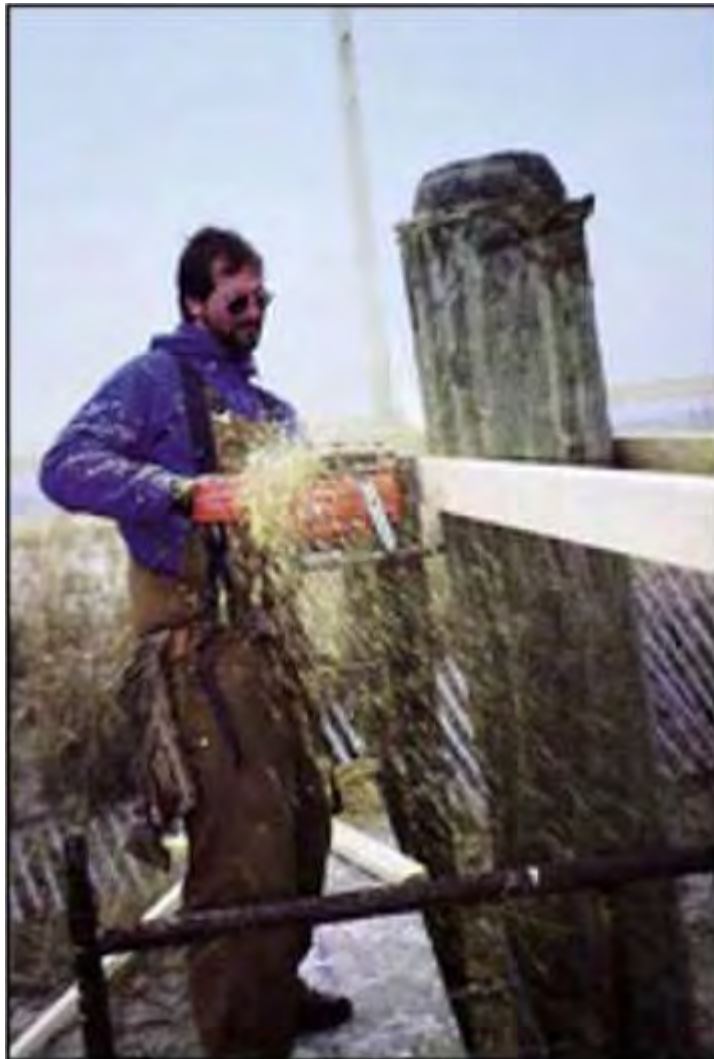
Figure 2. Typical pile notching process. Photograph by Patty McDaniel.
