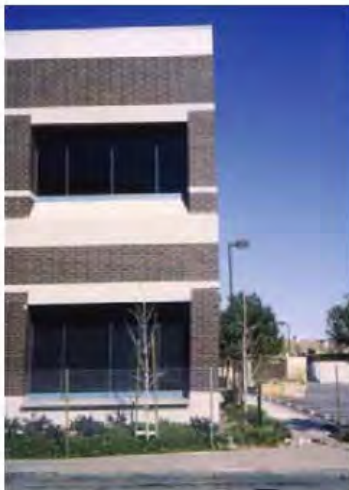
Figure 3: An example of a recently designed building with seismic deficiencies not understood at the time of design. In this case, the deficiency was "pre-Northridge" moment-frame connections, which proved to be extremely brittle and unsatisfactory. Hundreds, if not thousands, of these buildings were designed and built in the two decades before the Northridge earthquake (1994).
