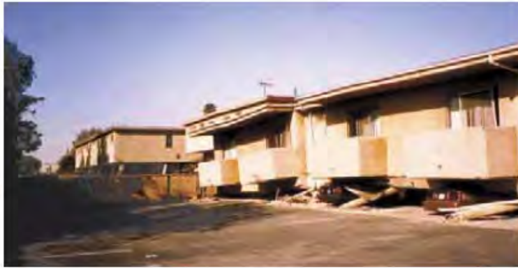
Figure 4: A 1970s building type with a deficiency not prohibited by the code at the time—a tuck-under apartment with parking at the ground level, creating a weak story. Many of these buildings collapsed in the Northridge earthquake. Sixteen deaths occurred in the Northridge Meadows apartments, or 42% of those directly killed by the earthquake.
