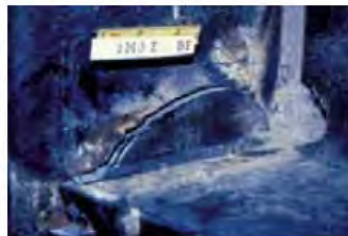
Figure 3: An example of a recently designed building with seismic deficiencies not understood at the time of design. In this case, the deficiency was "pre-Northridge" moment-frame connections, which proved to be extremely brittle and unsatisfactory. Hundreds, if not thousands, of these buildings were designed and built in the two decades before the Northridge earthquake (1994).
