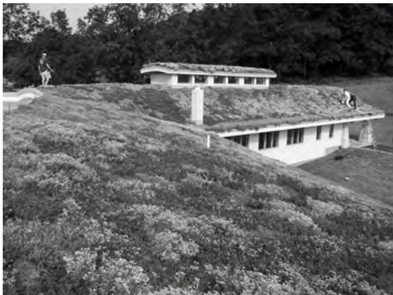
An extensive green roof by Charlie Miller, Roofscapes, Inc., for the Chiropractic Life Expression Wellness Center in Sugar Loaf, Pennsylvania.
